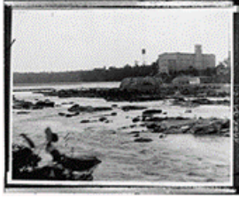
Bibb Company (Columbus Plant), Thirty-eighth Street & First Avenue (Columbus vicinity), Columbus, Muscogee County, GA Library of Congress, Prints and Photographs Division, HAER GA, 108-COLM,27-
